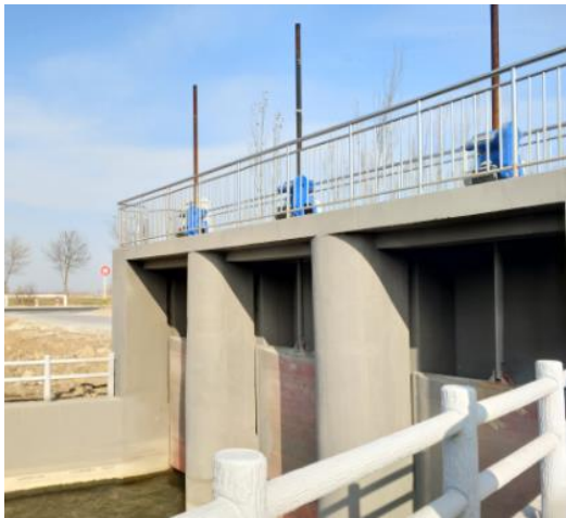
渠扩鱼池出水闸
