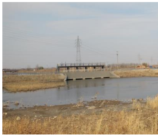
跨黄河节制闸
