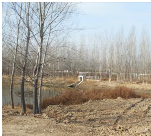
鱼池支渠 2 节制闸
