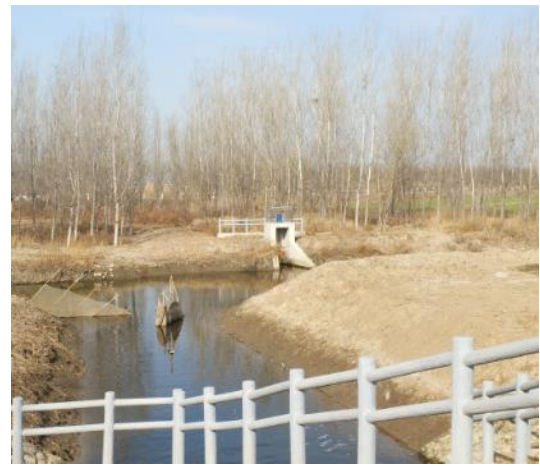
鱼池支渠 1 节制闸
